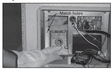
Figure 6.8 Place & Fasten Junction Box
